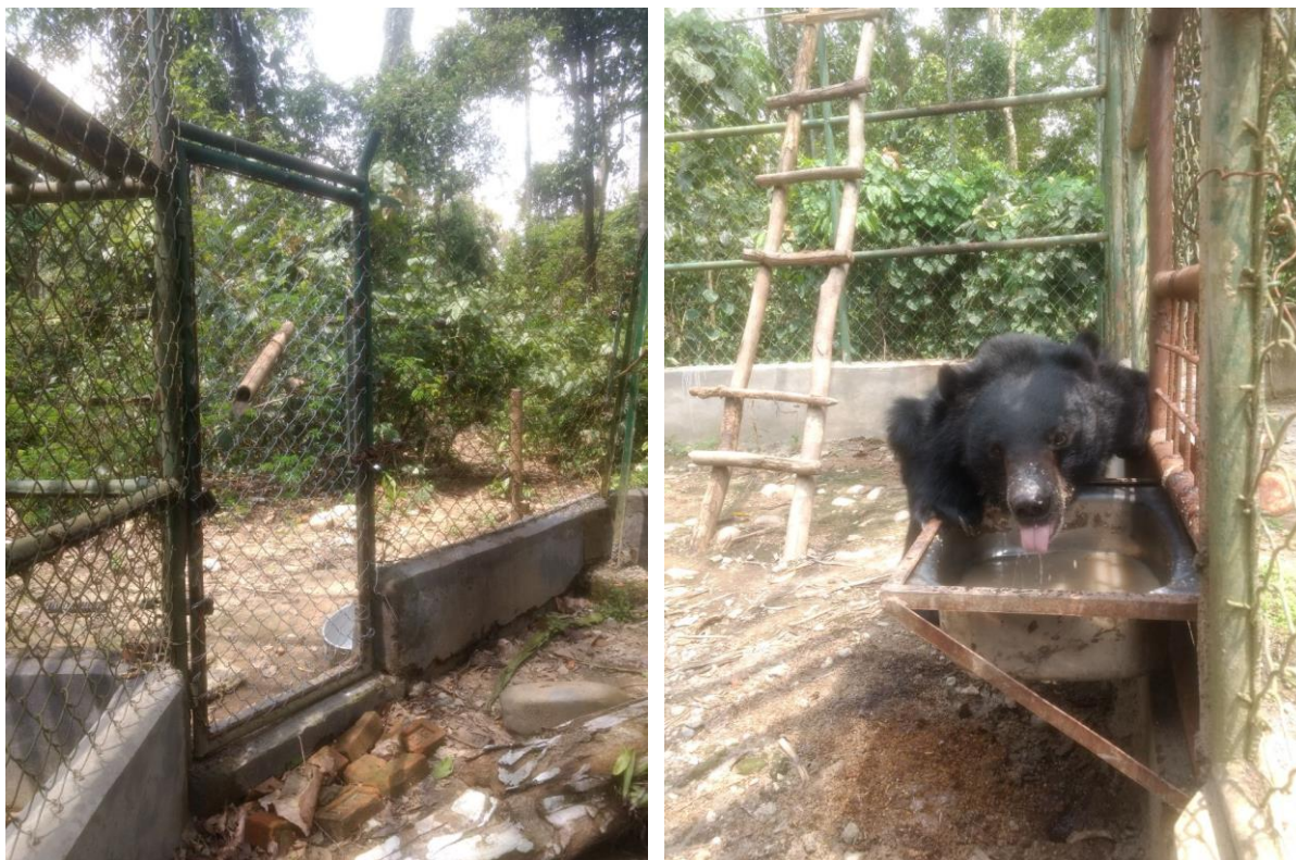
(L) Reinforced chain-link mesh and reconstructed foundation; (R) Bear lapping water from the newly constructed water trough
